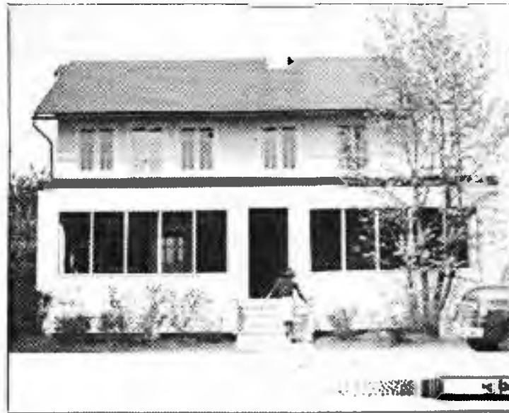
The St. Joan's House, the home of Miss Elisabeth Port and her five adopted children, is one of the last remaining structures of what was known as Childerley. The park district plans to demolish it.
