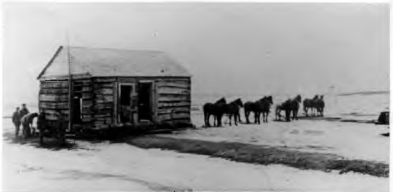
SMALL LOG CABIN BEING MOVED ACROSS PASTURE. BUILT IN 1835 - FIRST USED AS A HOME - LATER A PIG BARN. WAS TO BECOME 1ST CHAPEL AT CHILBERLEY - MOVED IN 1910..
