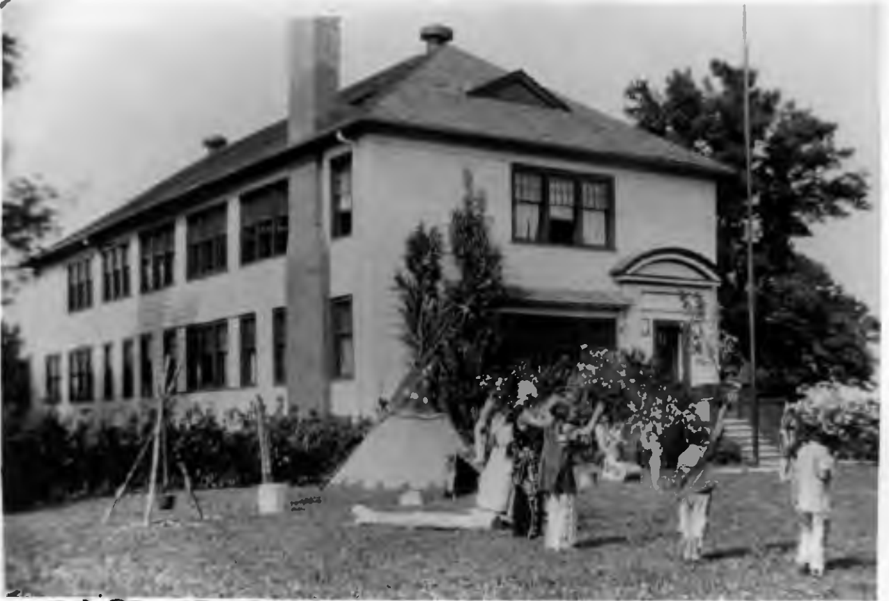
ON SITE OF NORTH FARM HOUSE (NOW PART OF VILLA BLOGS)
