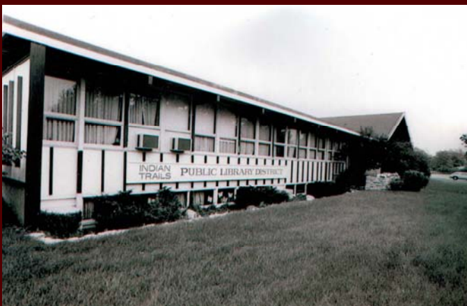
3rd location of Wheeling Library Formerly St. Marks Church.
